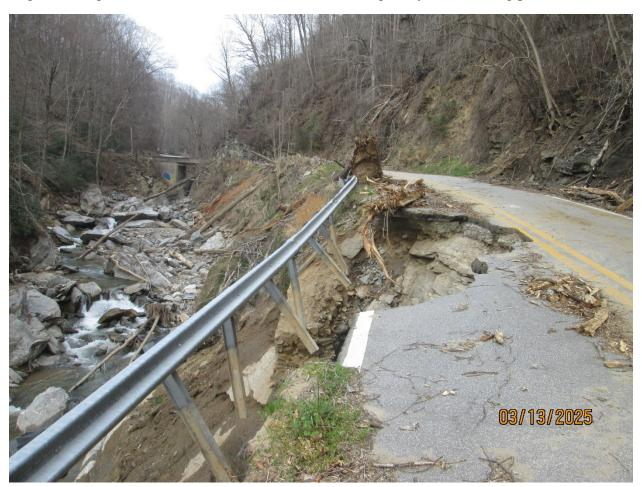
(Figure 1 – Typical Flood Damage to US 176)
