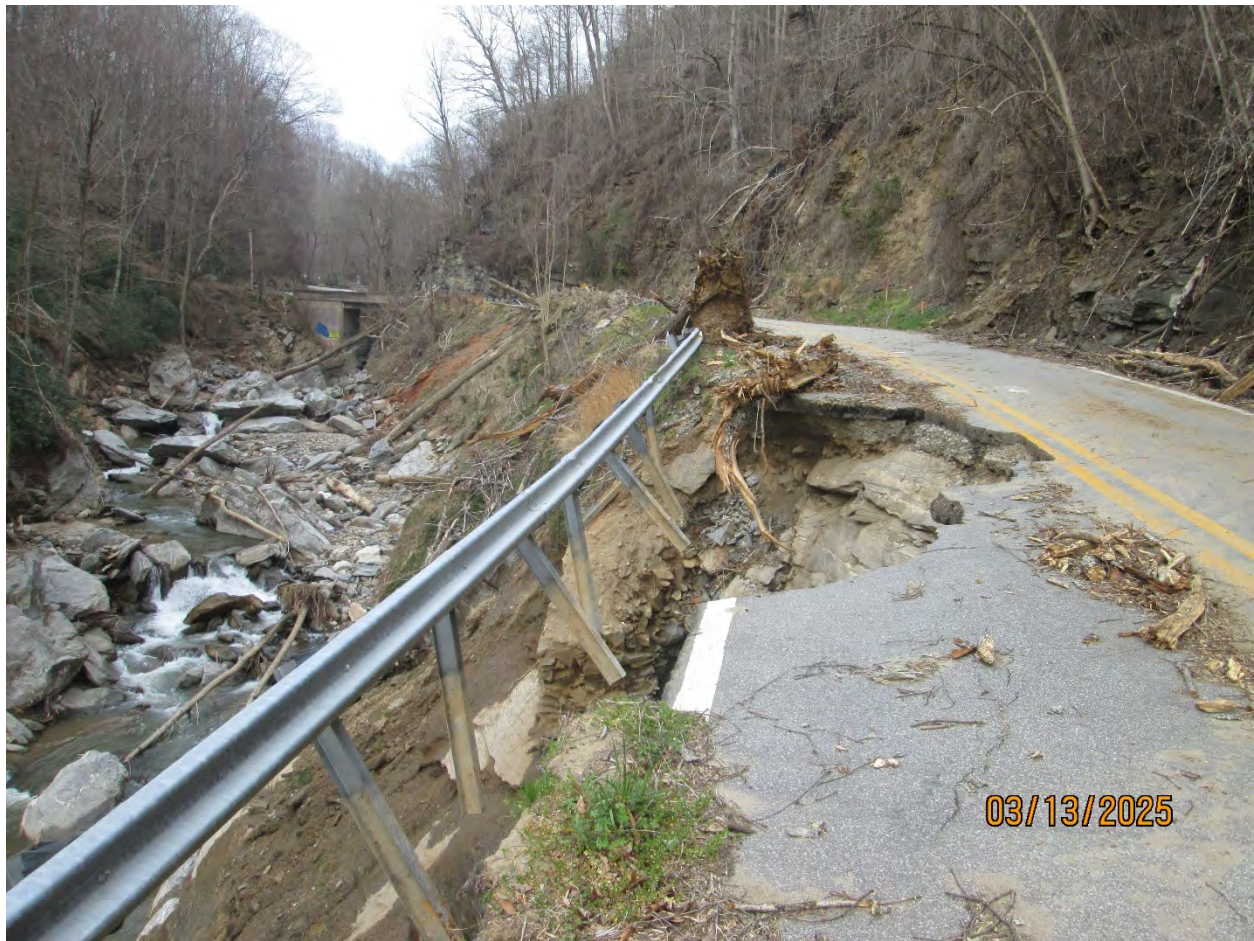
(Figure 1 – Typical Flood Damage to US 176)
