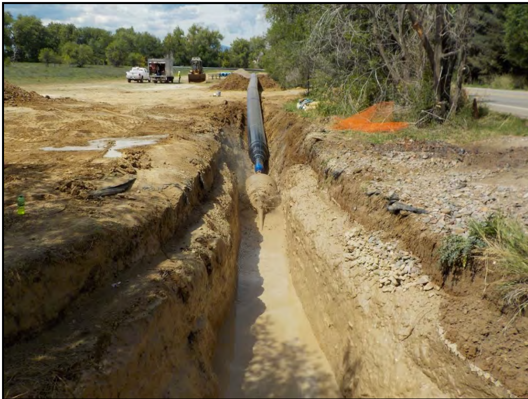
Figure 2 - HDD pit and pipe installation
