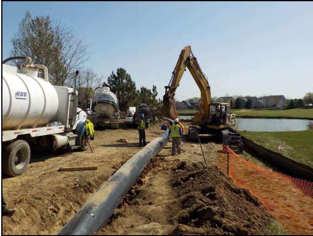
Figure 1 – HDD preparation
